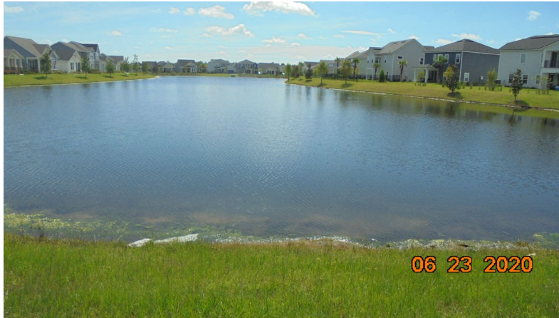
Pond 7c: Pond was a 7 (good condition). Water level is normal.
