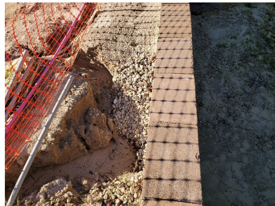
Image 16 – Monitoring of minor erosion
