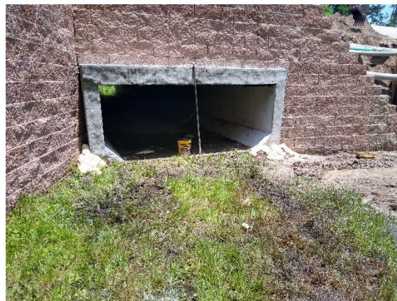
Image 4 – Filling of voids, Animal Crossing Box Culvert
