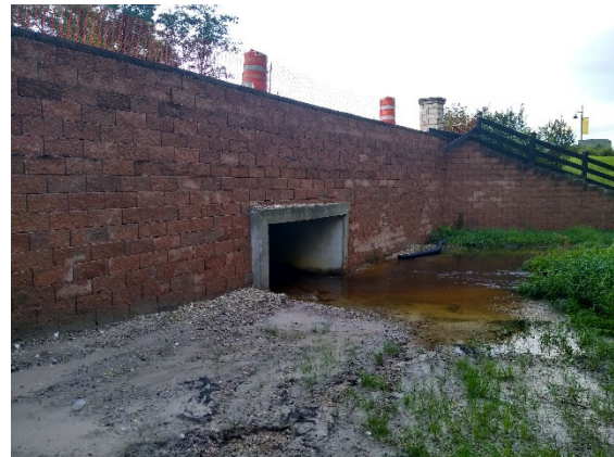
Image 12 – Repaired retaining wall
