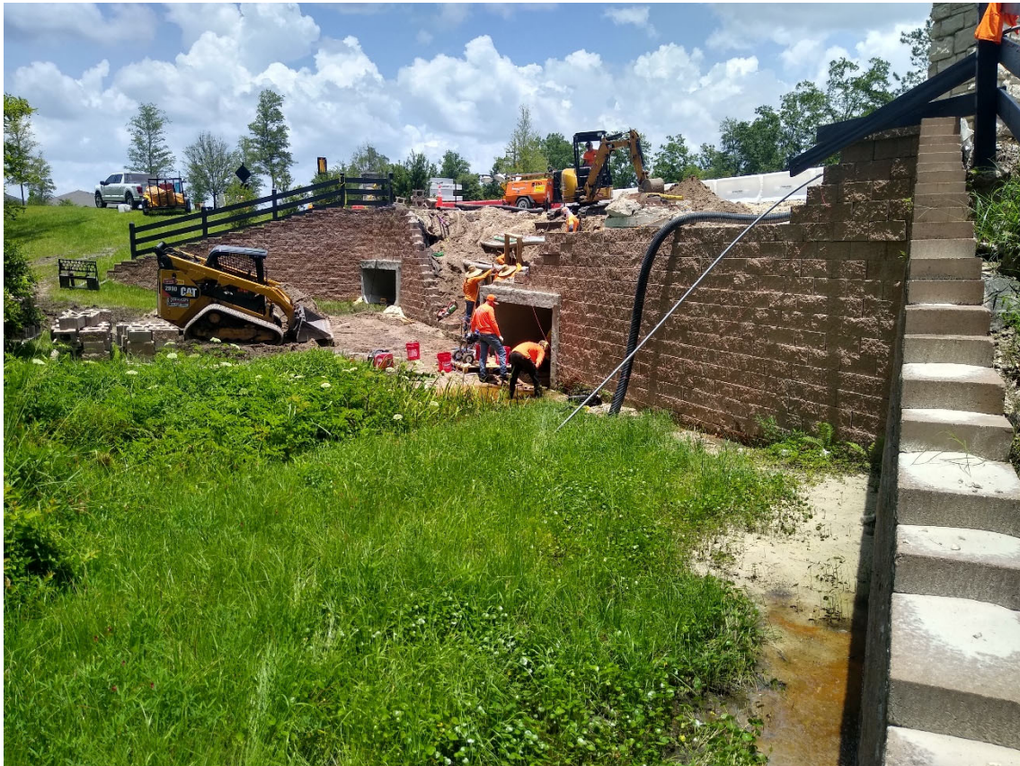
Retaining Wall View (Image 1)
