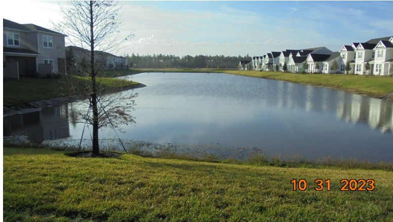
Pond 34: Pond was in good condition. The water level is good.
