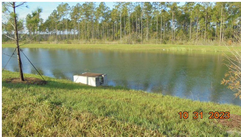
Pond 24b: Pond was in good condition.
