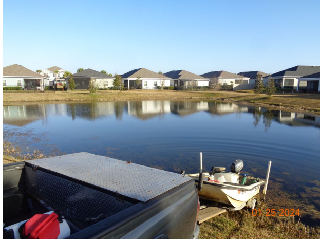
Pond 11b: Pond was in good condition. The water level is good.
