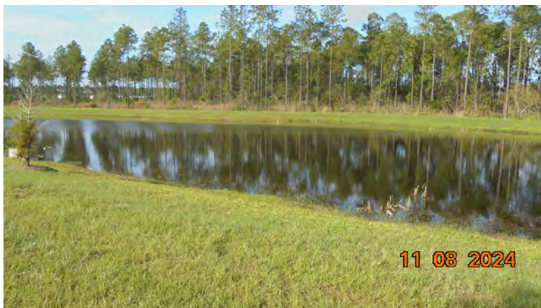
Pond 24a: Pond was in fair to good condition. Pond level is good. Perimeter treatment last month for cattails and torpedo grass was effective.
