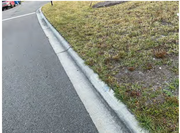
Concrete curb and gutter
