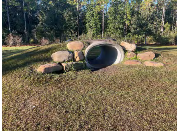
Dog park concrete tunnel
