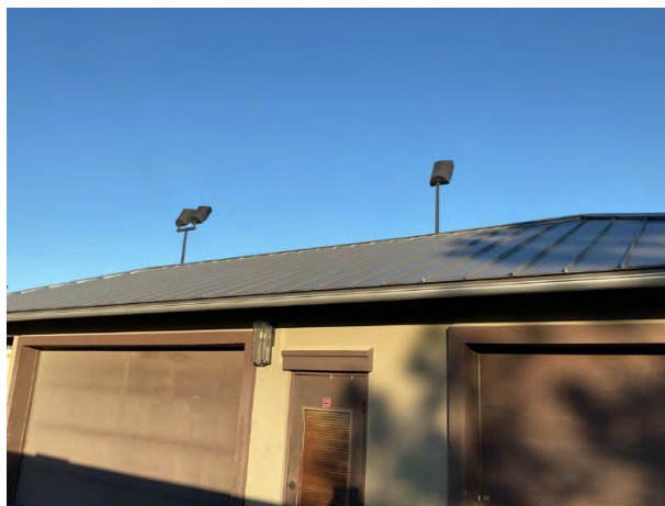
Metal roof overview at the Maintenance Building
