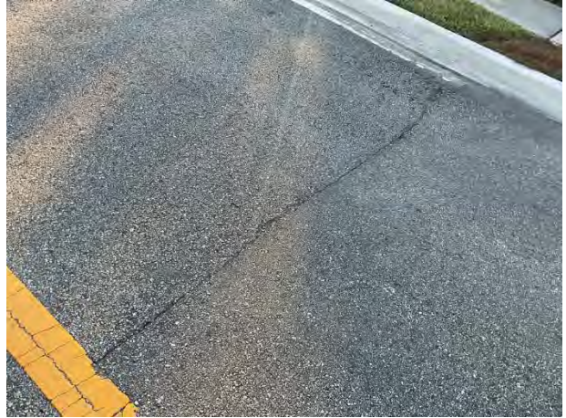
Pavement cracks
