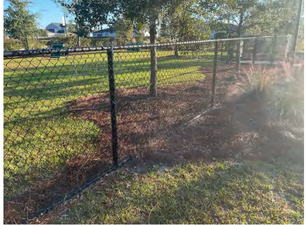
Chain link fence
