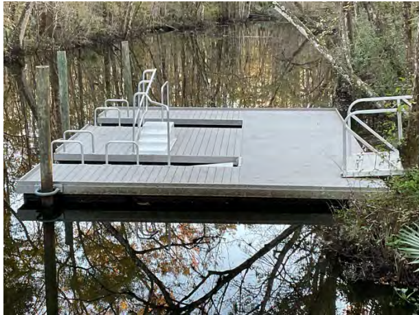
Dock with composite decking
