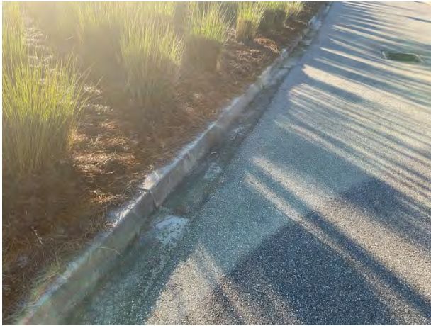
Concrete curb and gutter
