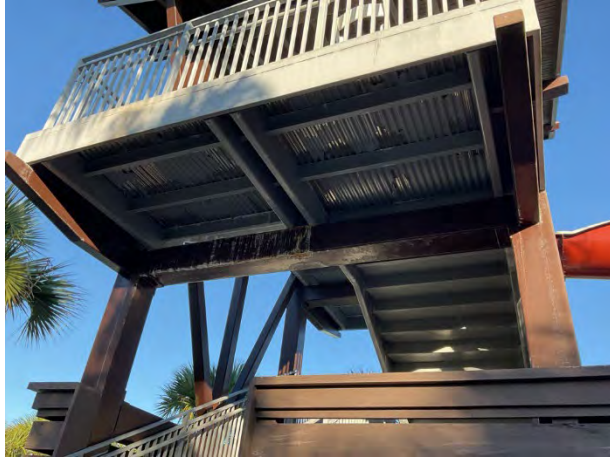
Staircase and balcony structure
