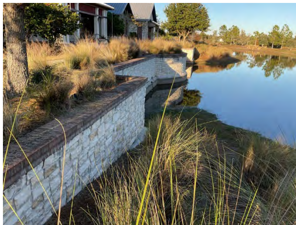
Stone bulkhead overview
