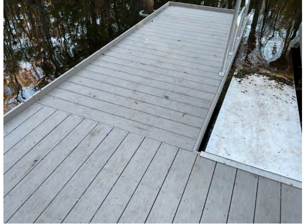
Dock with composite decking
