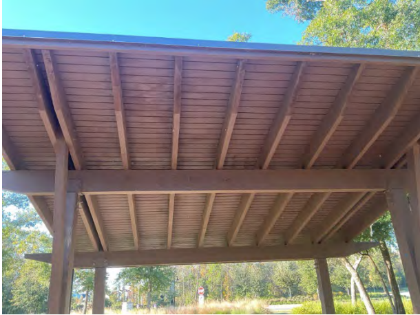
Pergola roof underside
