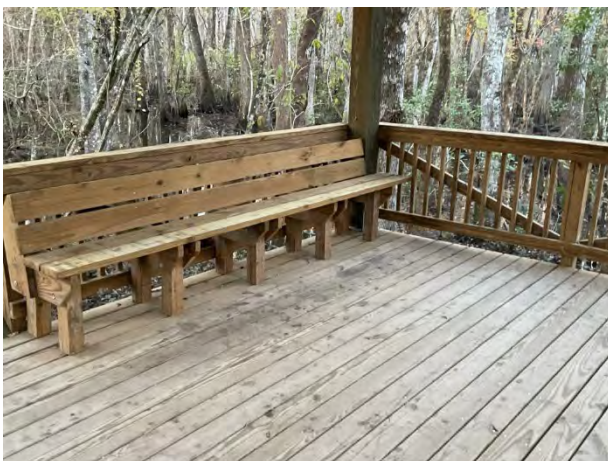
Dock with wood decking
