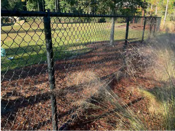
Chain link fence
