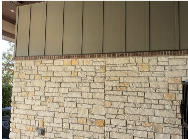
Masonry walls overview
