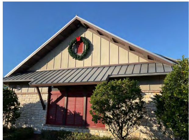
Metal roofs overview at Fitness Center
