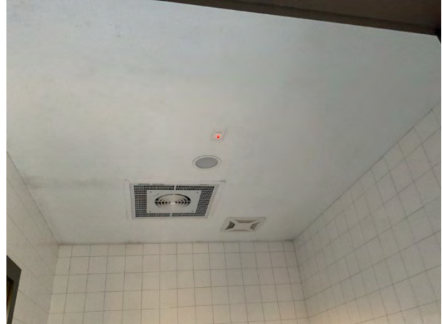
The Outpost rest room overview
