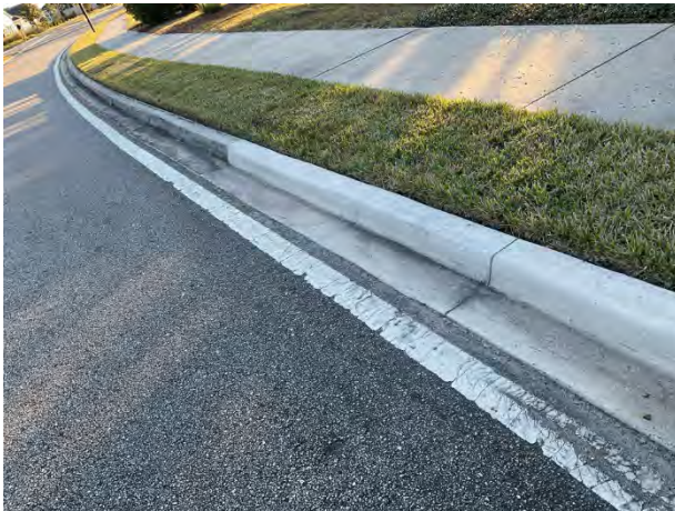
Concrete curb and gutter
