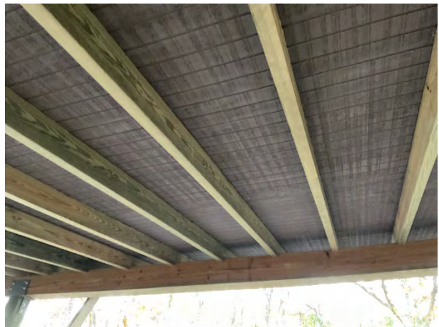
Pergola roof underside
