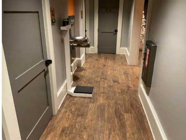
Vinyl floor covering at hallways
