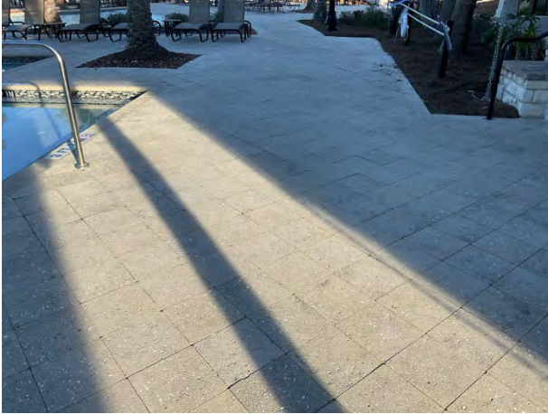
Paver pool deck overview
