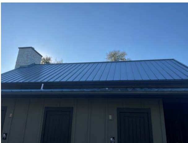
Metal roofs overview at the Outpost
