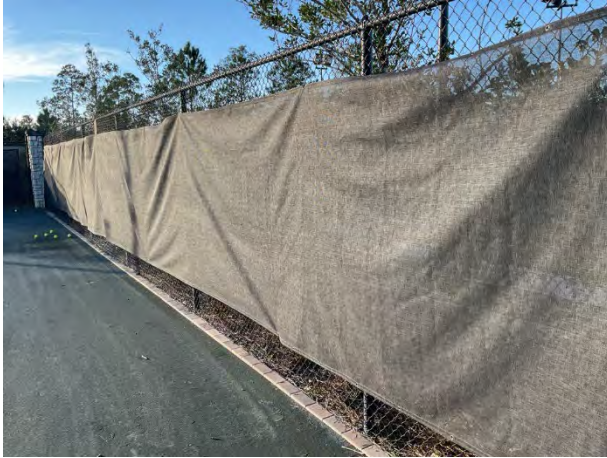
Chain link fence
