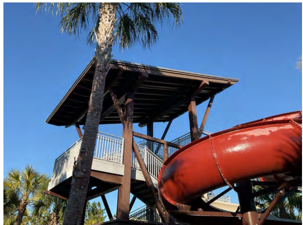
Metal roof at pool water slide
