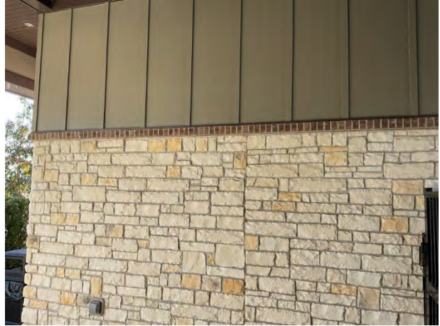
Masonry walls overview
