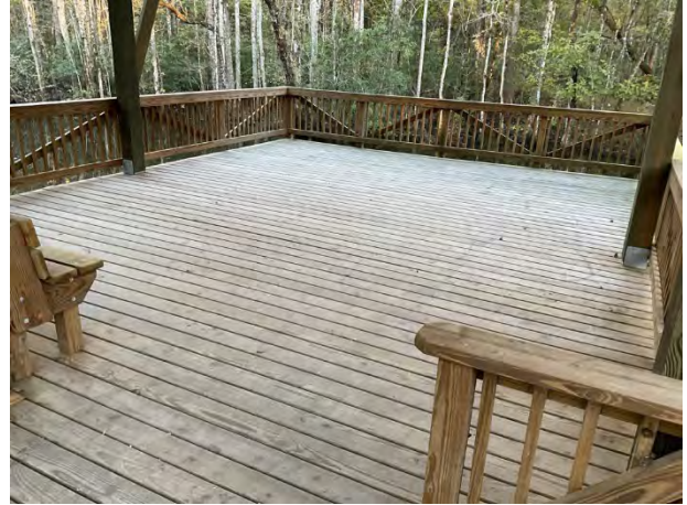
Dock with wood decking
