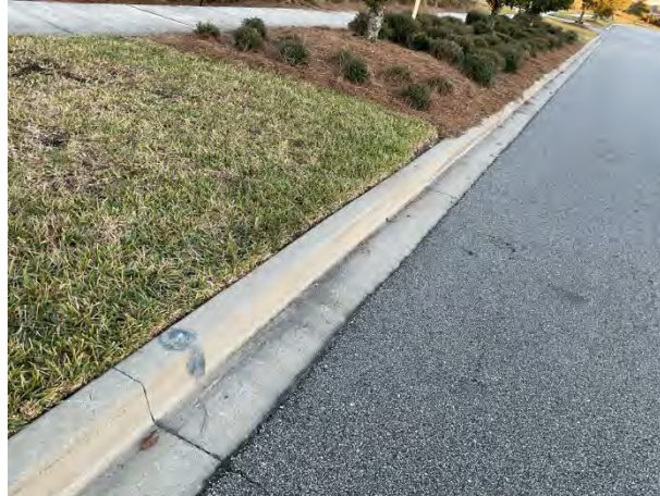
Concrete curb and gutter
