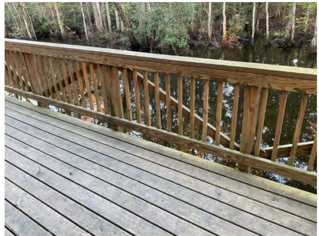
Dock with wood decking
