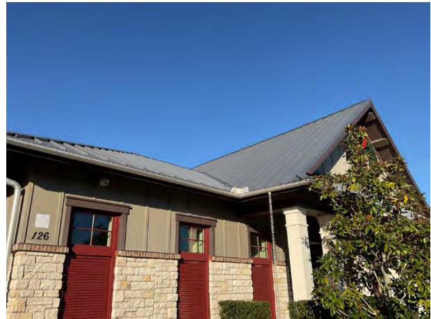
Metal roofs overview
