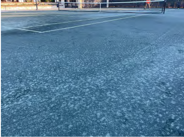
Tennis court overview
