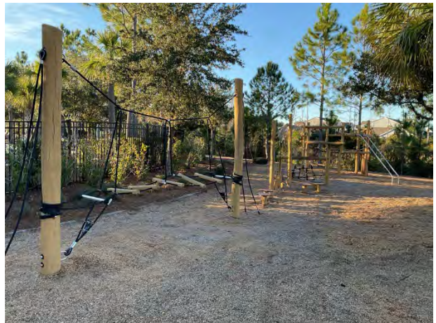
Playground equipment overview
