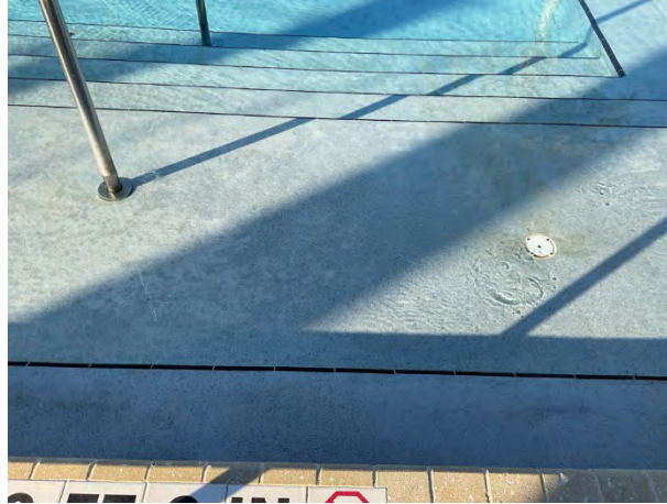
Lap pool plaster finish with tile perimeter
