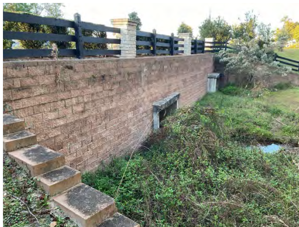
Masonry retaining walls overview
