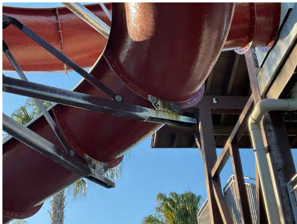
Rusted fasteners
