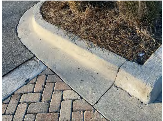
Concrete curb and gutter
