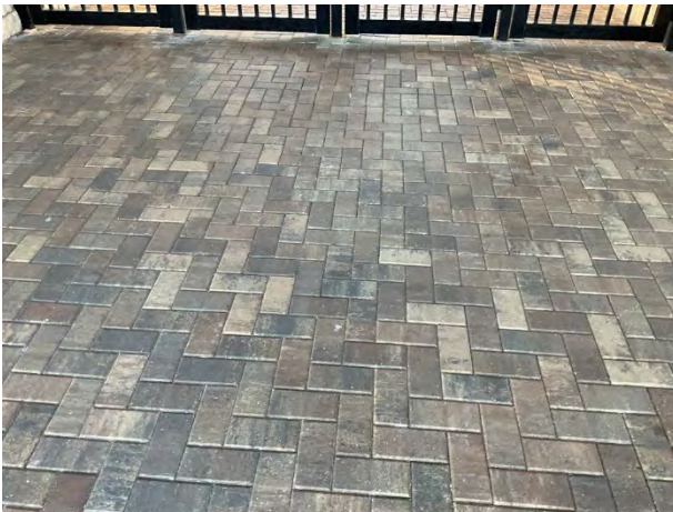
Paver pool deck overview
