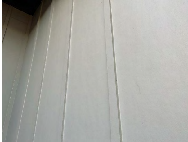
Fiber cement siding overview
