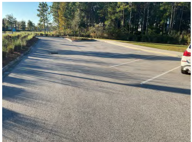
Dog park pavement overview
