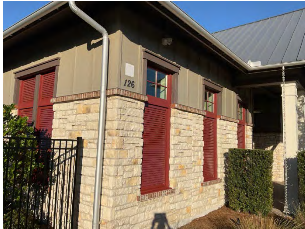
Masonry walls overview
