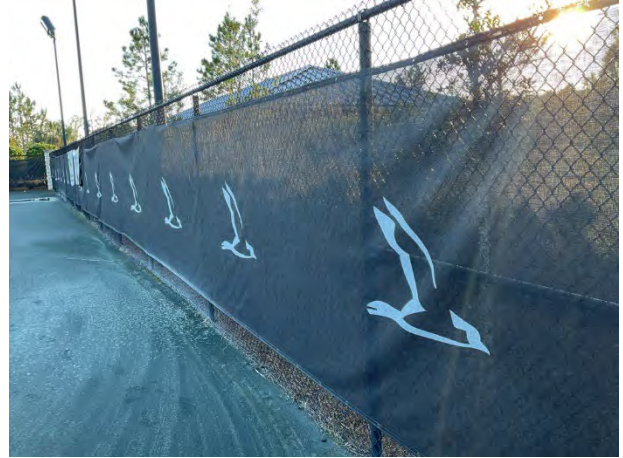
Chain link fence
