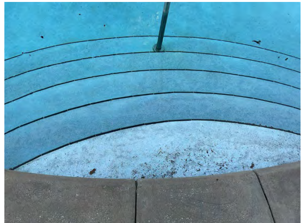
Lazy River plaster finish with tile perimeter
