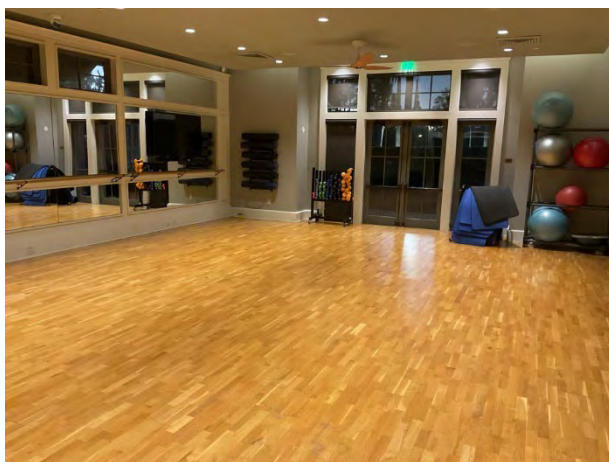
Vinyl floor covering at yoga room
