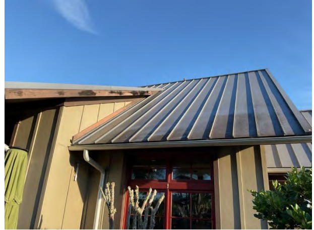
Metal roofs overview at Fitness Center
