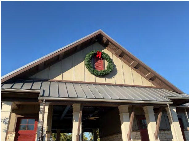
Metal roof overview
