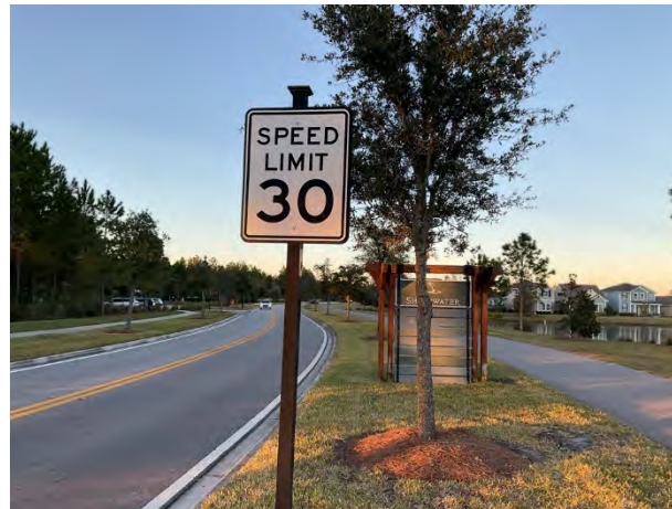
Traffic management signage
