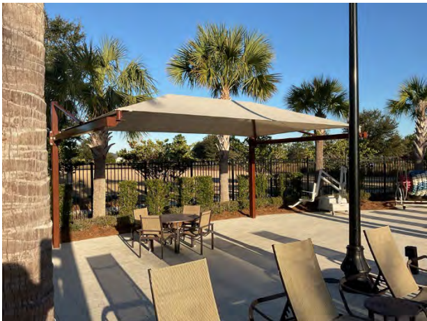
Shade structure at pool area
