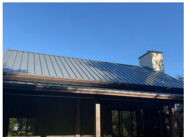
Metal roofs overview at the Outpost
