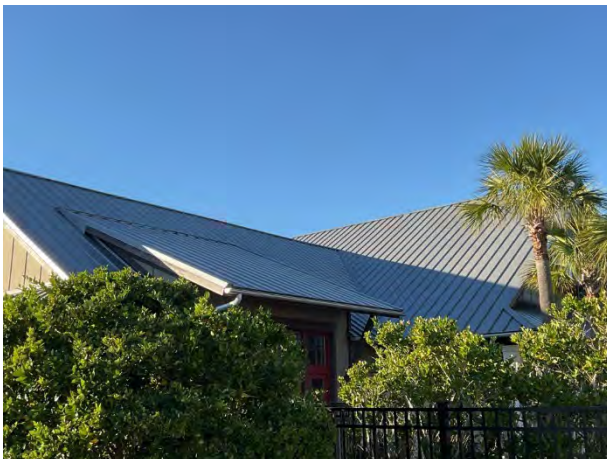
Metal roofs overview at Fitness Center
