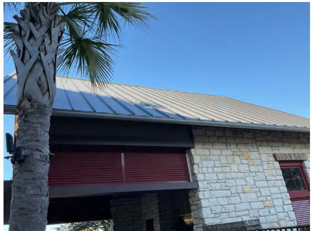
Metal roof overview at the Party Pavillion
