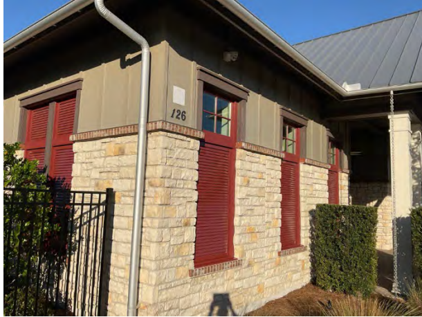
Masonry walls overview
