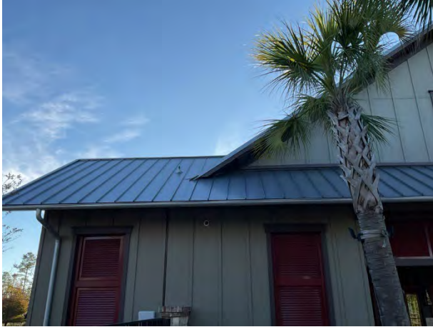
Metal roofs overview at Fitness Center
