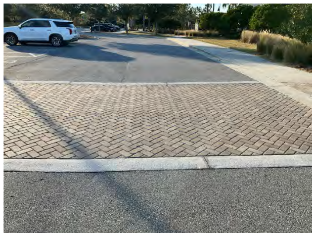
Parking area pavement overview
