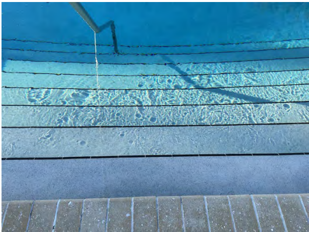
Main pool plaster finish with tile perimeter
