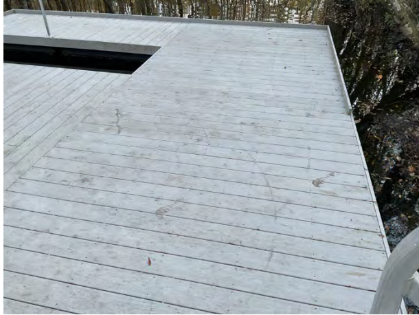
Dock with composite decking
