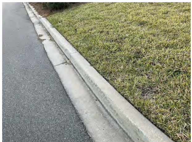
Concrete curb and gutter
