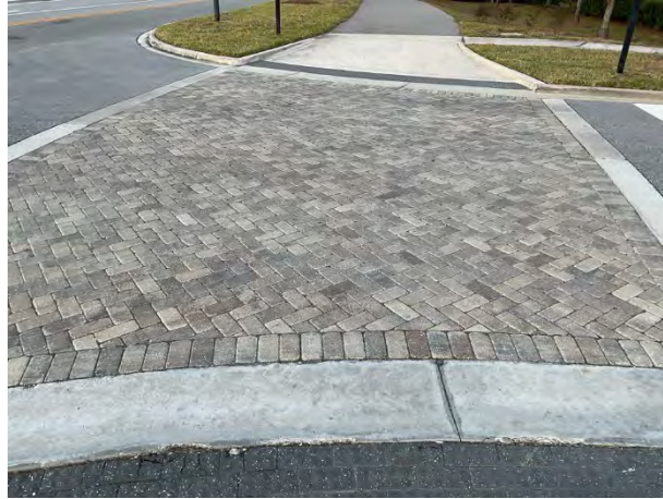
Masonry pavers overview
