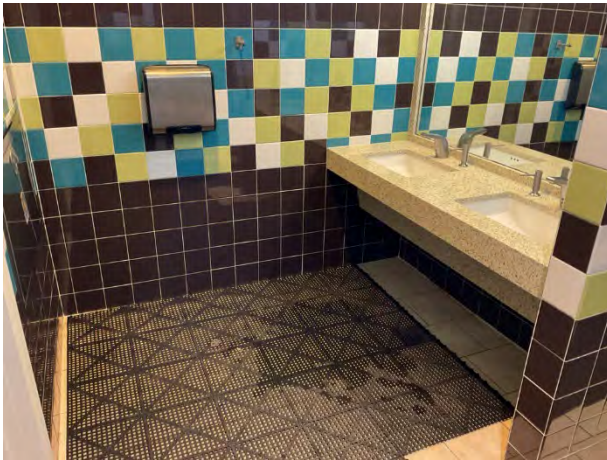
Rest room overview
