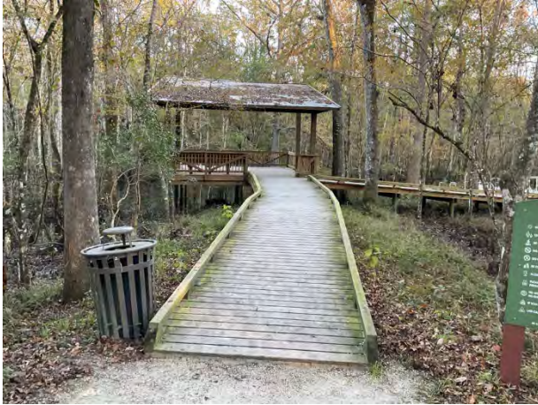
Wood docks overview
