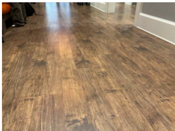
Vinyl floor covering at lobby
