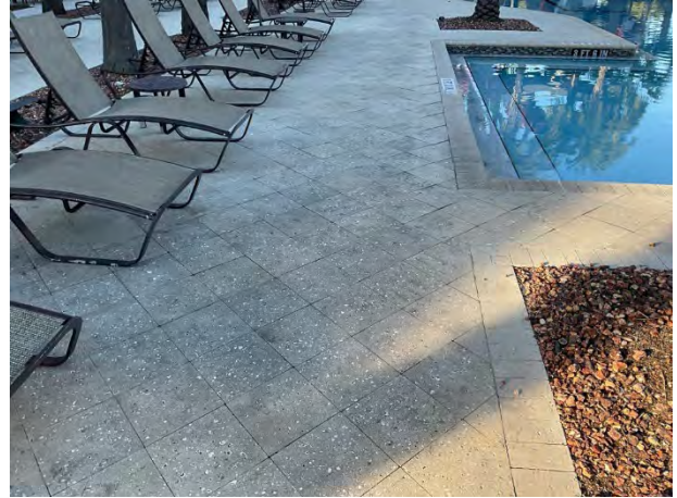
Paver pool deck overview
