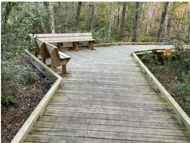
Boardwalk overview with wooden benches
