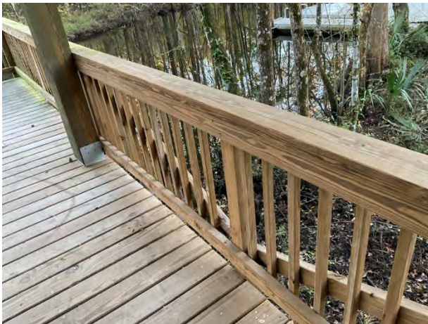
Dock with wood decking
