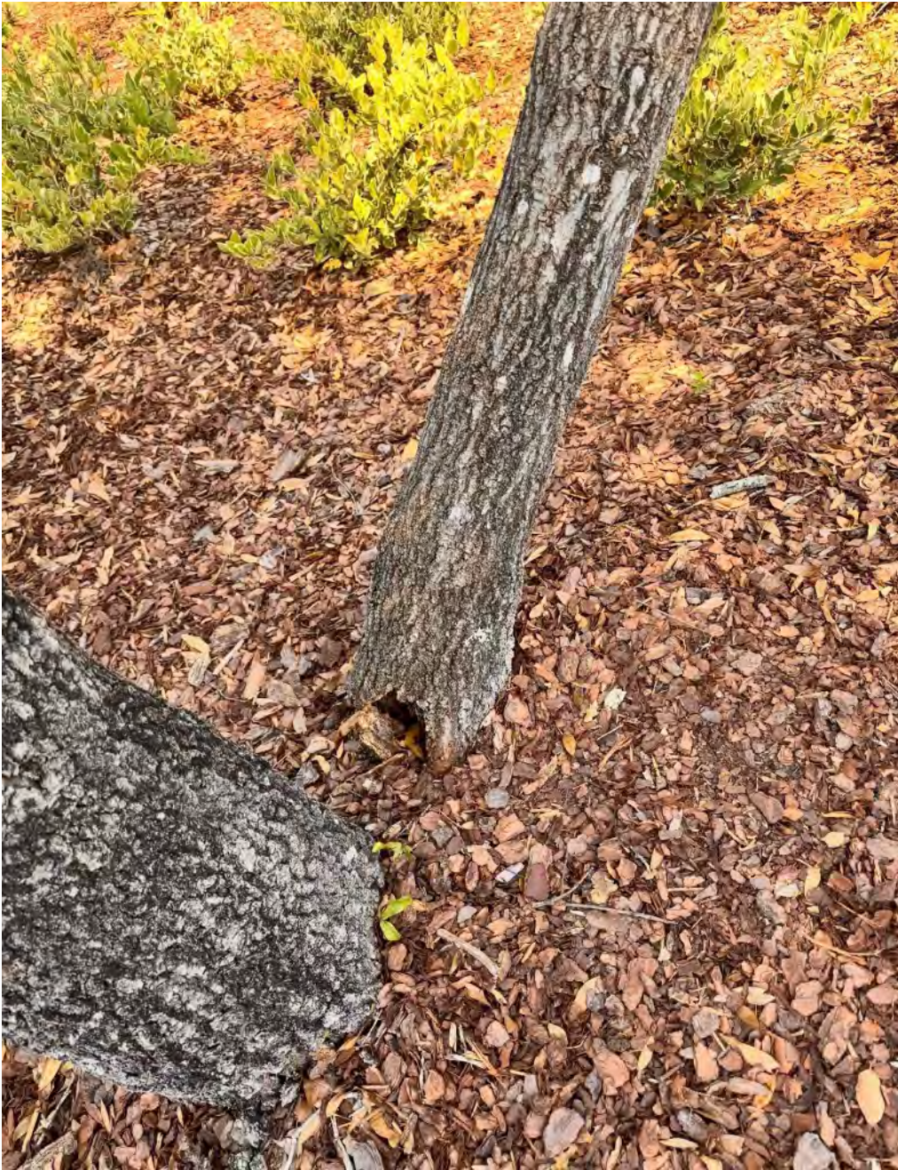
Falling Tree At Kayak Outpost Will Be Removed By Shaw Tree Service Created: Fri, 4/4/2025
