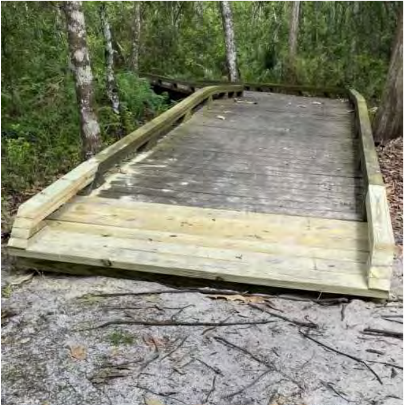
Repaired Boardwalk Landing At Trail 9
