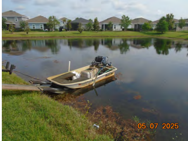
Pond 11b: Pond was in good condition. The water level is good. Perimeter treatment last month was effective.
