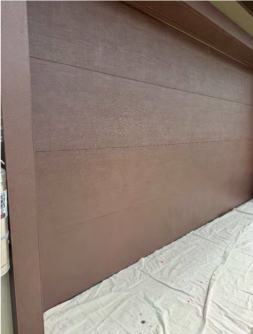
Painted Garage Doors At Maintenance And Lifestyles Storage.
