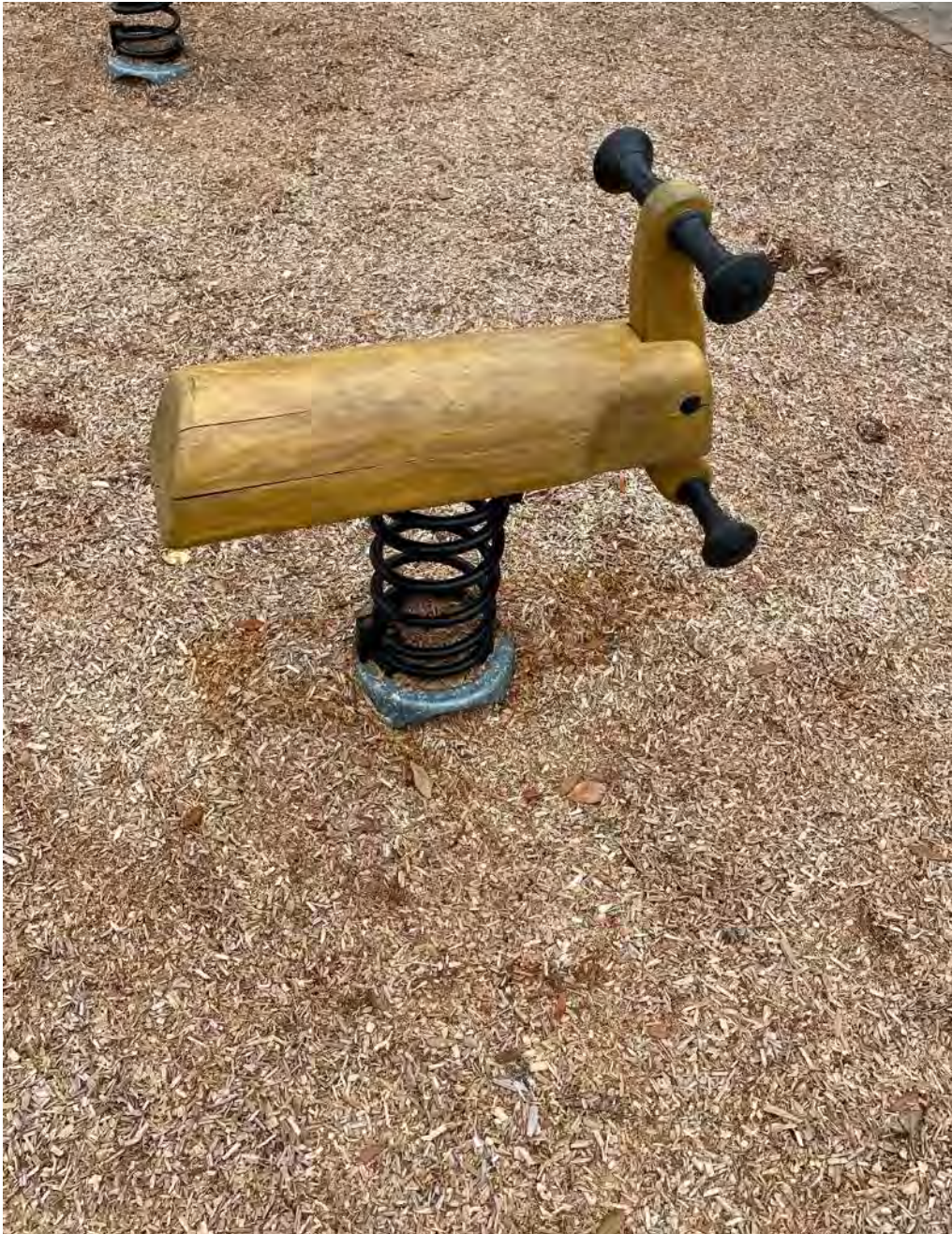
Stained Faded Play Equipment.
