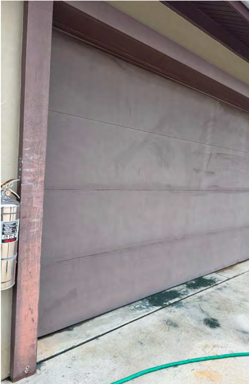
Painted Garage Doors At Maintenance And LifeStyles Storage.
