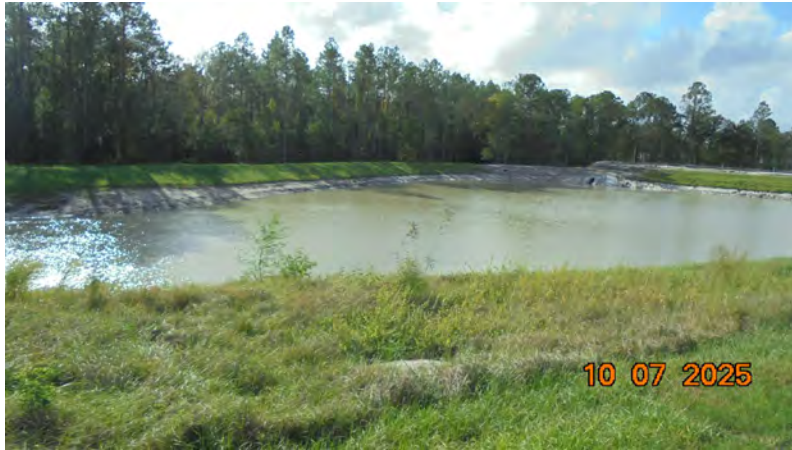
Pond 28A: Pond was in fair to good condition. The water level is good. Treated for cattails.
