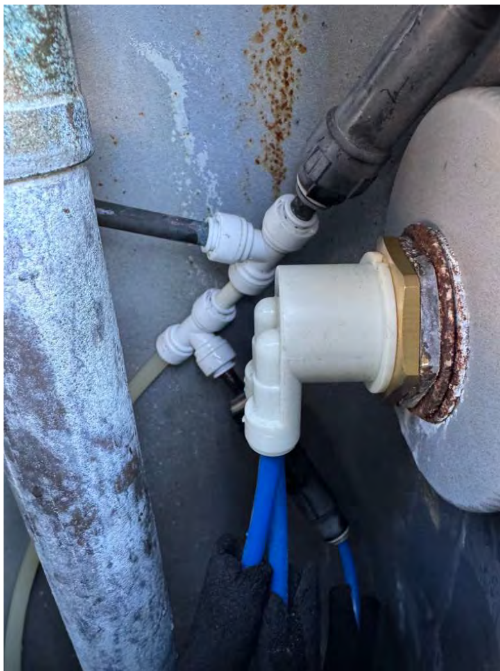
Replaced Broken Fountain Regulator At Dog Park.
